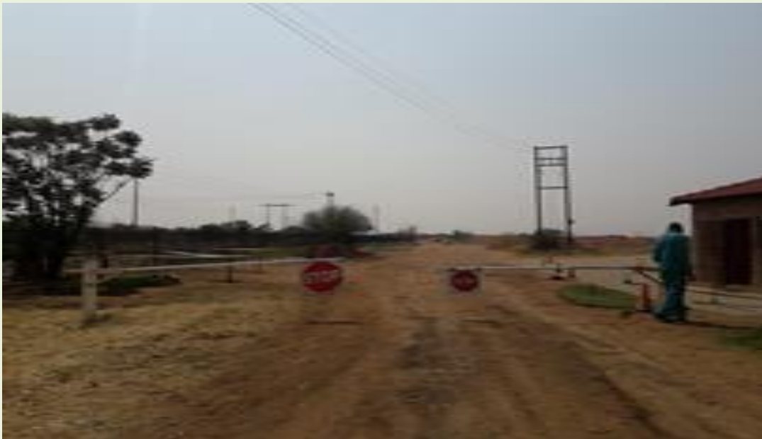
FIGURE:4 LANDFILL DISPOSAL AREA(BEFORE)
