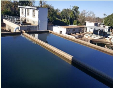
Bela- Bela Water Works
