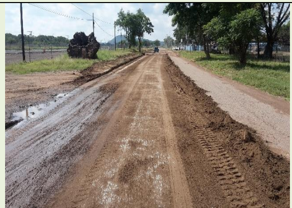
Grading of unpaved roads
