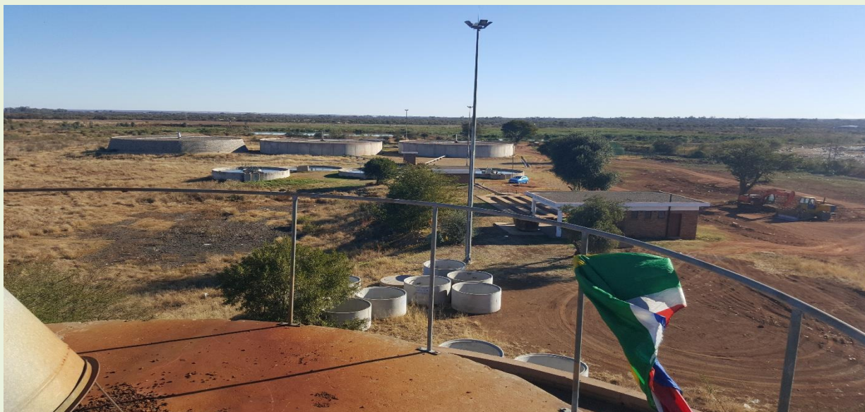
Warmbarths Waste Water Treatment Plant
