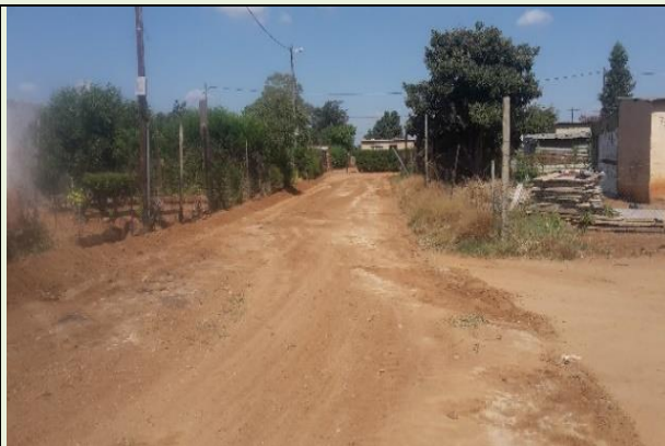
Routine road maintenance
